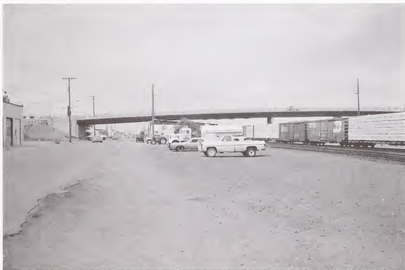
The Great Northern Railroad Overpass in Shelby. The structure is typical of many railroad overpasses constructed in Montana during the 1930s. The Commission constructed many overpasses to separate grade crossings for tracks and roads in an effort to reduce the number of railroad-related accidents.
